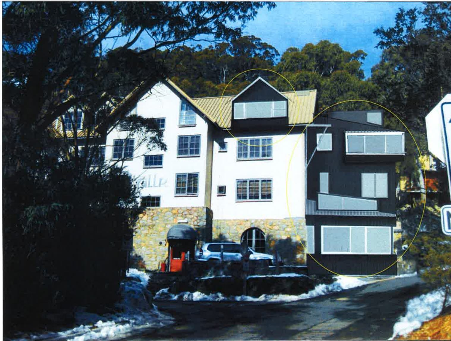
Figure 3: Photomontage of proposal looking towards the western façade of House of Ullr illustrating the new external additions and alterations (circled) (Source: Applicant's DA documentation)
